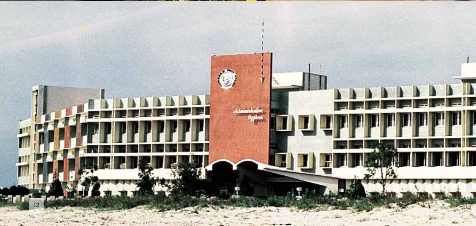
▲ LIC Regional Office, Madurai
