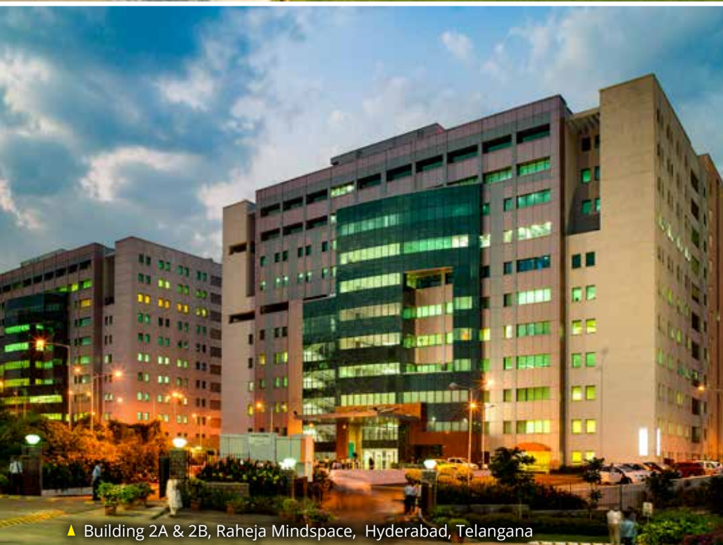
▲ Satyam IT Complex Phase I, Bahadurpally, Hyderabad, Telangana
