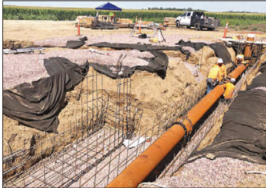
CONSTRUCTION ON Lewis & Clarks Rural Water System's million-gallon ground storage reservoir for Madison began construction in May. It's completion will signify the final piece of the puzzle for the city's full integration into the L&C system.
