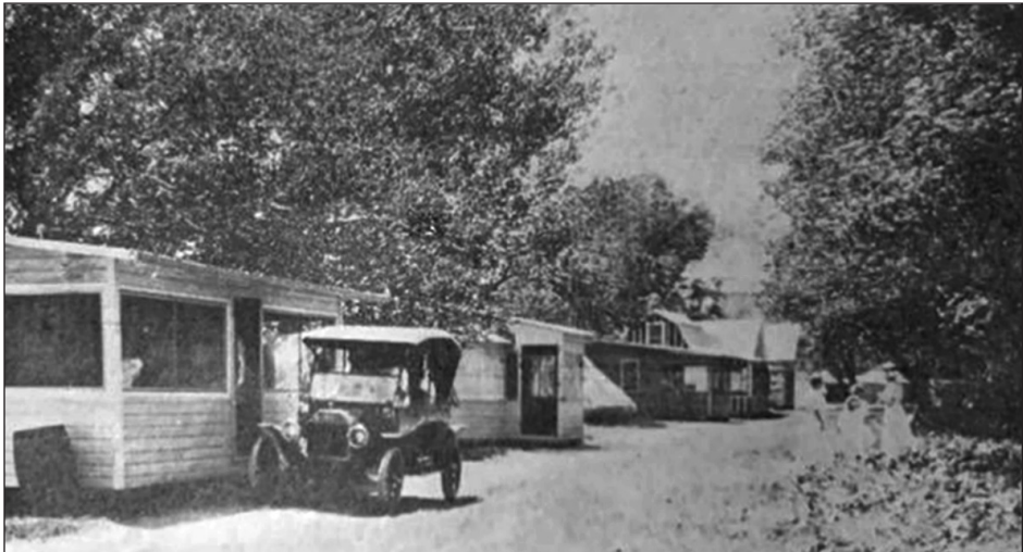
Cabins were added to provide additional lodging.
