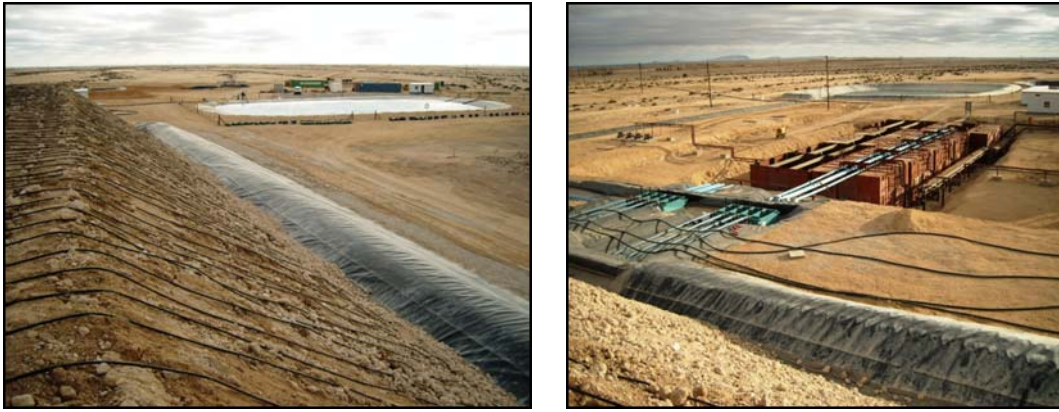
Plate 4.5: Trekkopje mini heap leach pad and storage tanks for the ‘pregnant leach’, during early trial stages of the mine design and construction in 2008 (photo Geological Survey).
