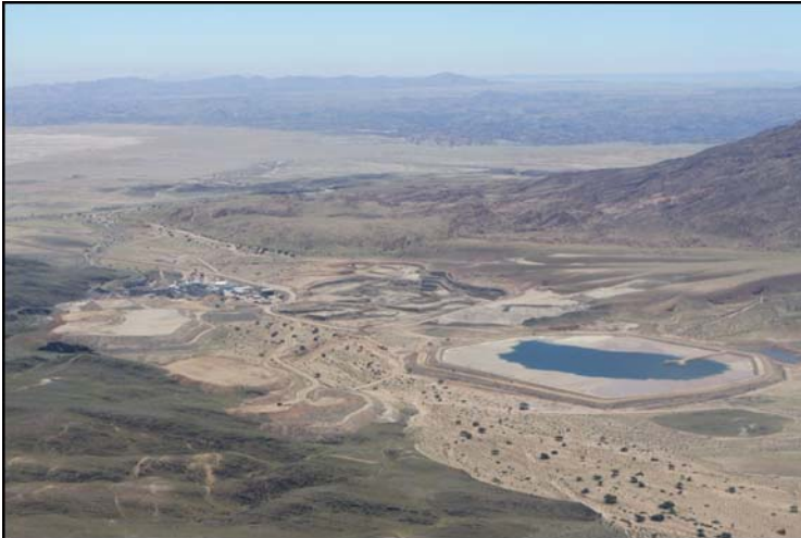
Plate 7.4.2: Tailings dams need to be carefully located, well designed and constructed, properly maintained and closed according to international best practice to avoid contamination of groundwater resources. The Langer Heinrich tailings dam is situated in a dry river channel, which could be hazardous in the event of a large flood (photo P.Tarr).
