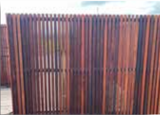
Kwila 1.8m vertical hit and miss screen fence and gate. Constructed from steel or timber frame with internal rails, clad with 32x32mm kwila batons with a 20mm gap between batons. Clad both sides.
