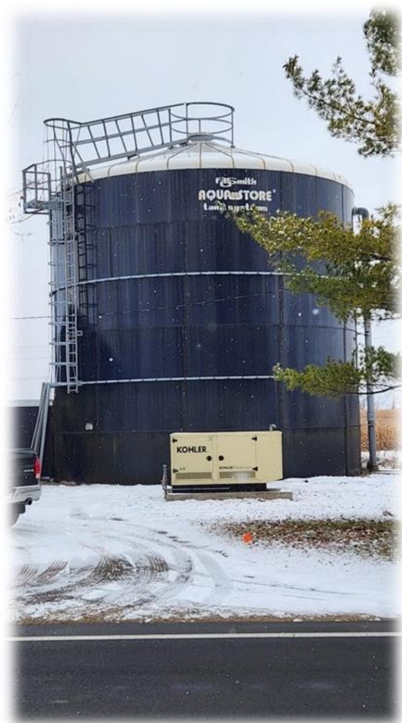
New Water Tower
