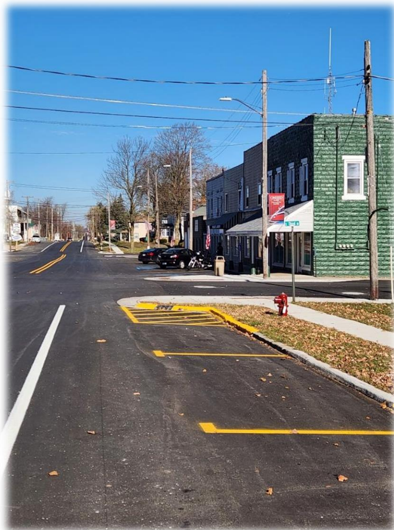
Street Paving Project, Downtown Onsted 2023
