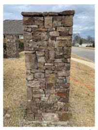
4. <u>Dimensions</u>: the columns must be 27" square (27" x 27"). Column height (including stone cap) must be 9" (nine inches) above the top of the ornamental fence (minimum height of ornamental fence facing a common area is six feet).
