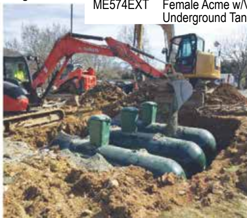
Backfill tanks ensuring 6" of sand around tanks.
