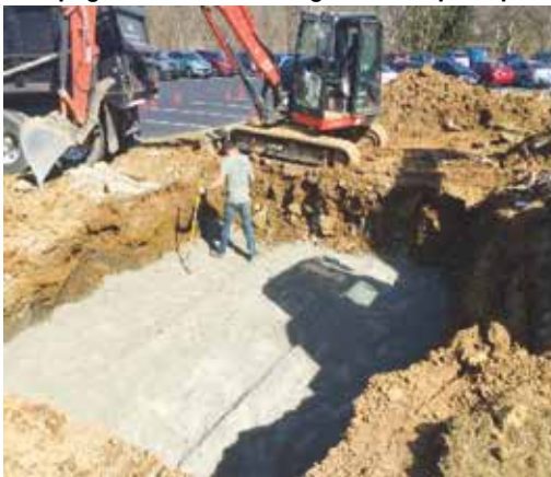
Place 6" of sand on bottom of hole.
