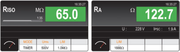
Measurement of insulation resistance.
