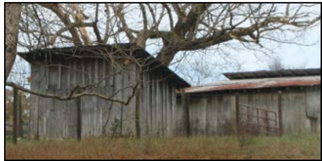
Larkins Farm barns, 2025. Photograph by author.
