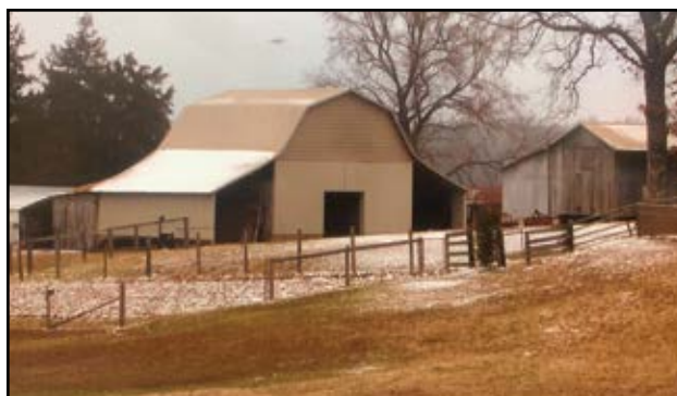
Bennett Farm, 2009. A 1940s barn covered in metal in 2002 by Gailford, Weldon, Burton, and Seth Bennett. Tennessee Century Farms Files.
