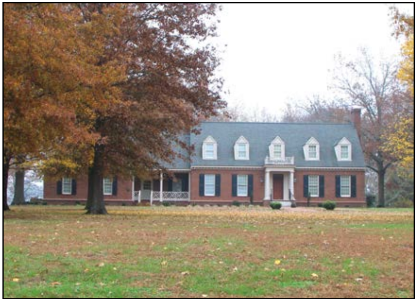
Allen Farm house, 2025. Photograph by the author.
