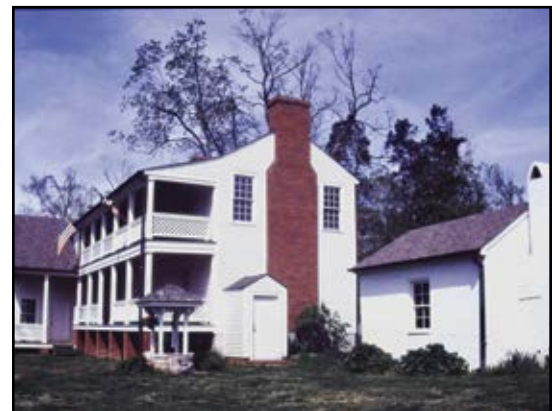
Woodard Hall Farm house, rear, 1994. Photograph by the author.
