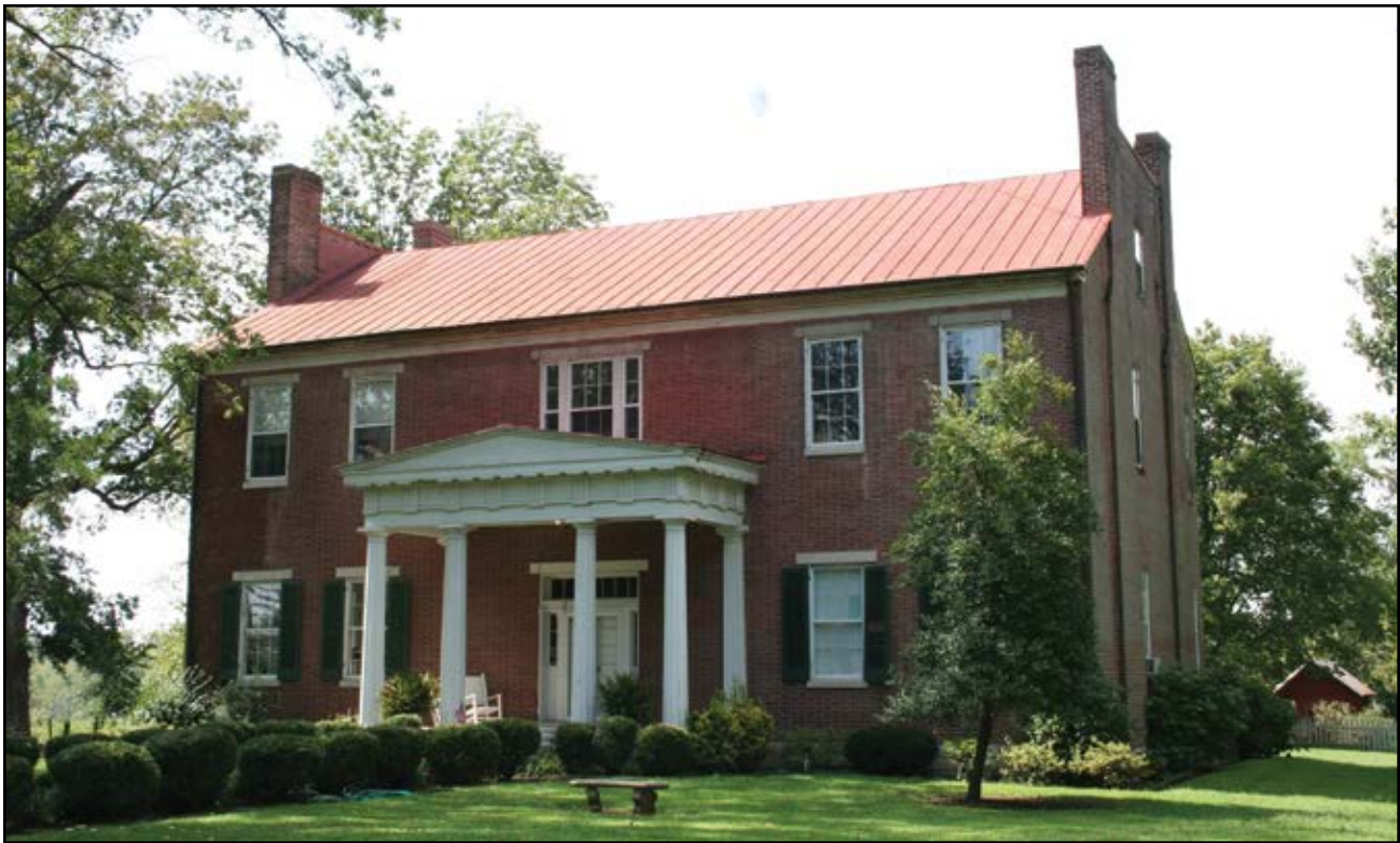
Cleveland Hall Farm. Metro Nashville Historical Commission.
