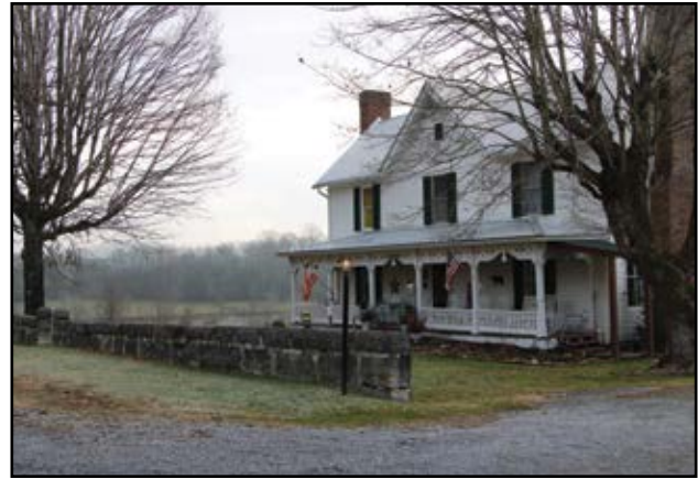
Brabson Ferry Farm historic house. Photograph by the author.
