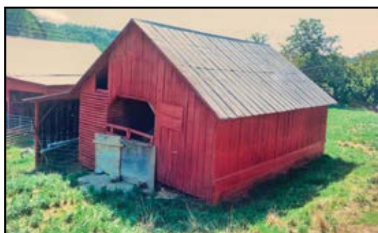
King Farms crib and granary. Tennessee Century Farms Files.
