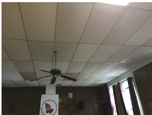
Detail of the dropped ceiling and fan, installed c. 1983-1988
