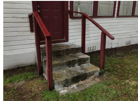
Detail of concrete steps, c. 1983
