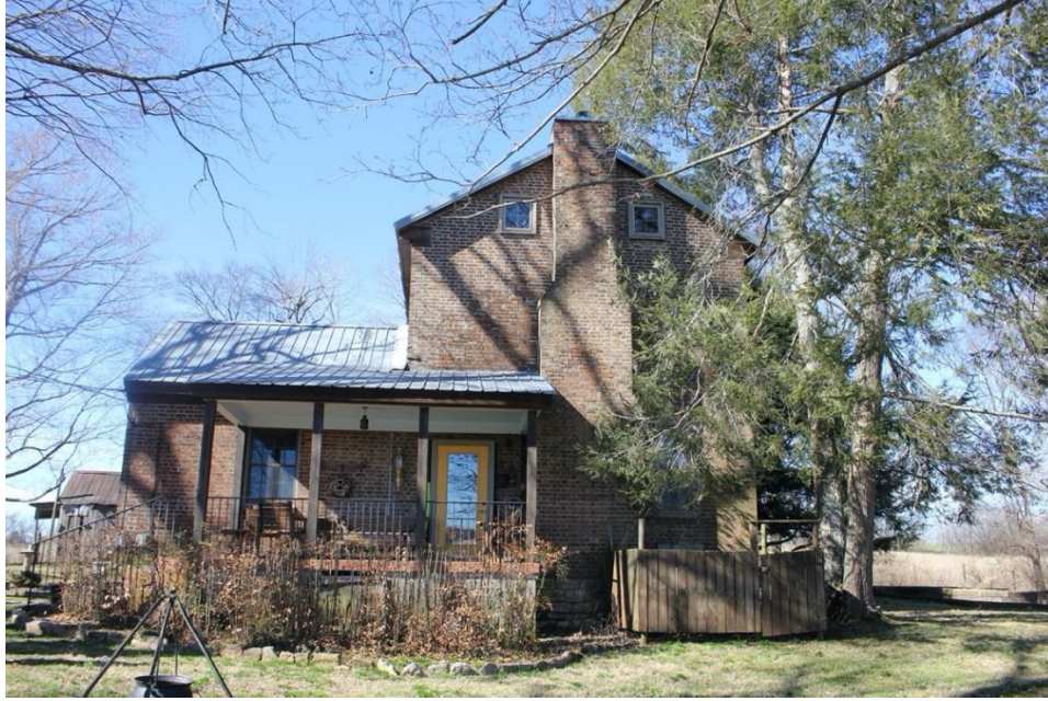
East elevation, February 2024.
