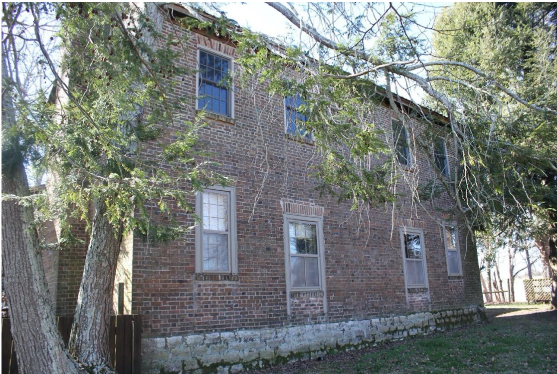
North elevation, February 2024.
