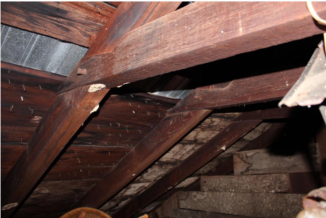
Hewn-and-pegged joint system visible in attic, February 2024.
