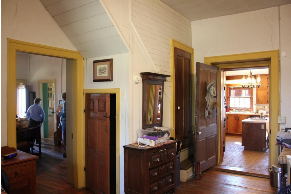
Enclosed stairway in west room leading to west side of second story, February 2024.
