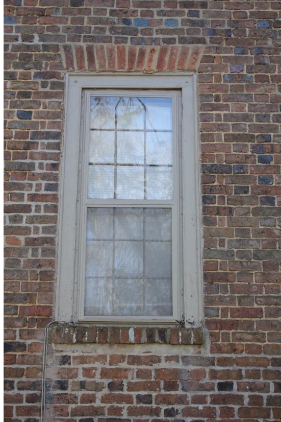
Flat lintels above window, February 2024.
