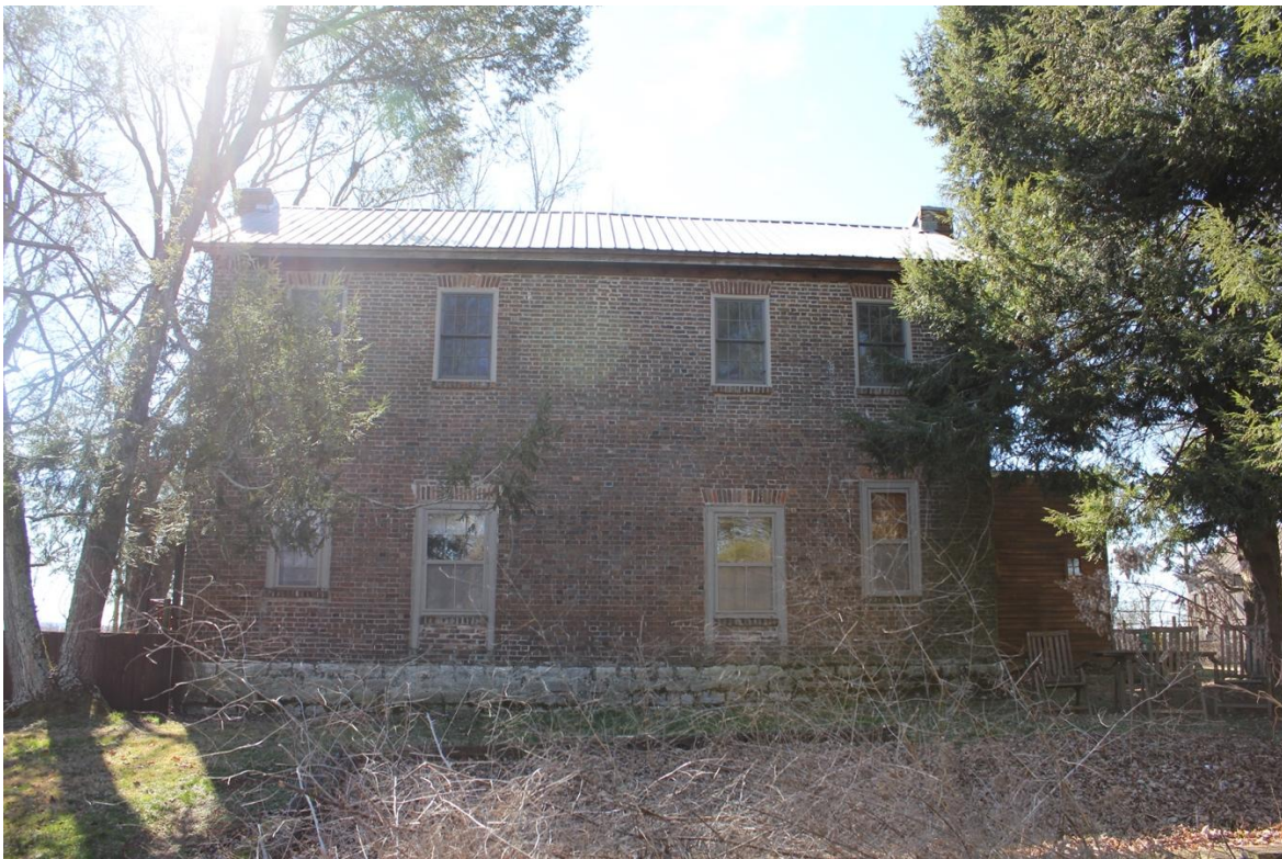
North elevation/original front of Matt Martin House, February 2024.
