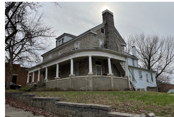
Figure 92. Rock House, 209 West Main St.
