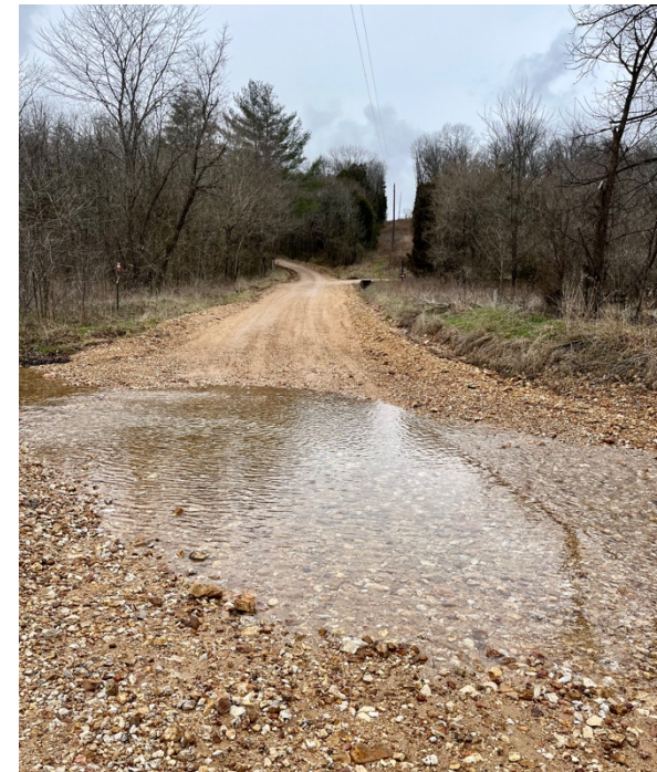
Figure 11. Original road segment through the Brickey Farmstead site.
