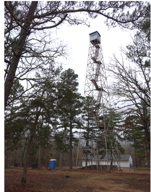
Figure 110. Marcoot Fire Lookout Tower.
