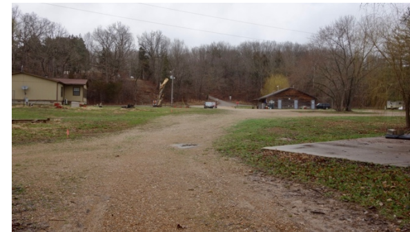
Figure 24. Looking north towards Spring Rd. with the convenience store on the right.
