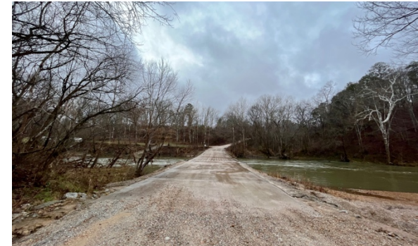
Figure 76. Boiling Springs Road/Mo-BB, looking southwest.
