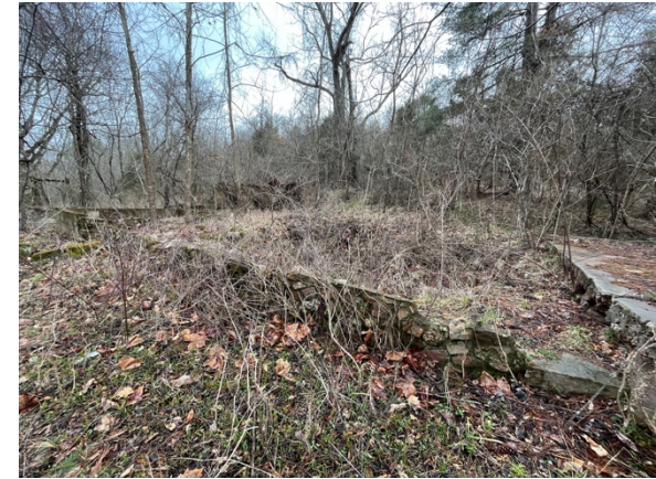
Figure 10. Brickey House foundations.
