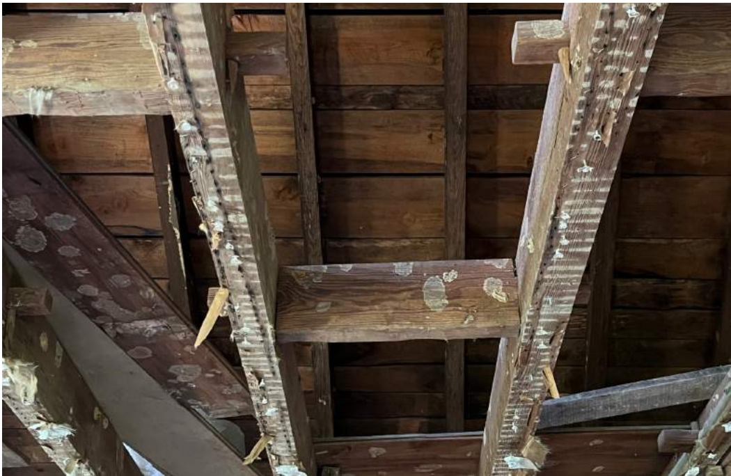
Figure 9. Examples of wood pegging in the house, 2022.
