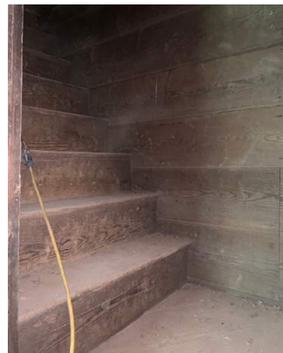
Figure 17. Box stairs detail, 2022.
