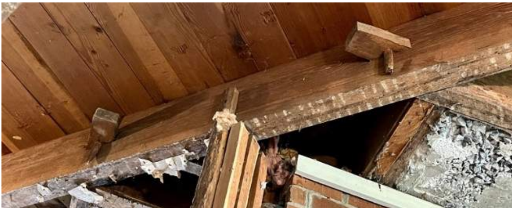
Figure 10. Examples of wood pegging in the house, 2022.
