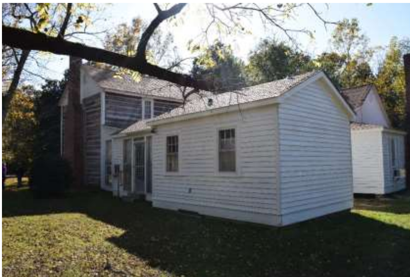
Figure 6: 1960s bathroom addition.
