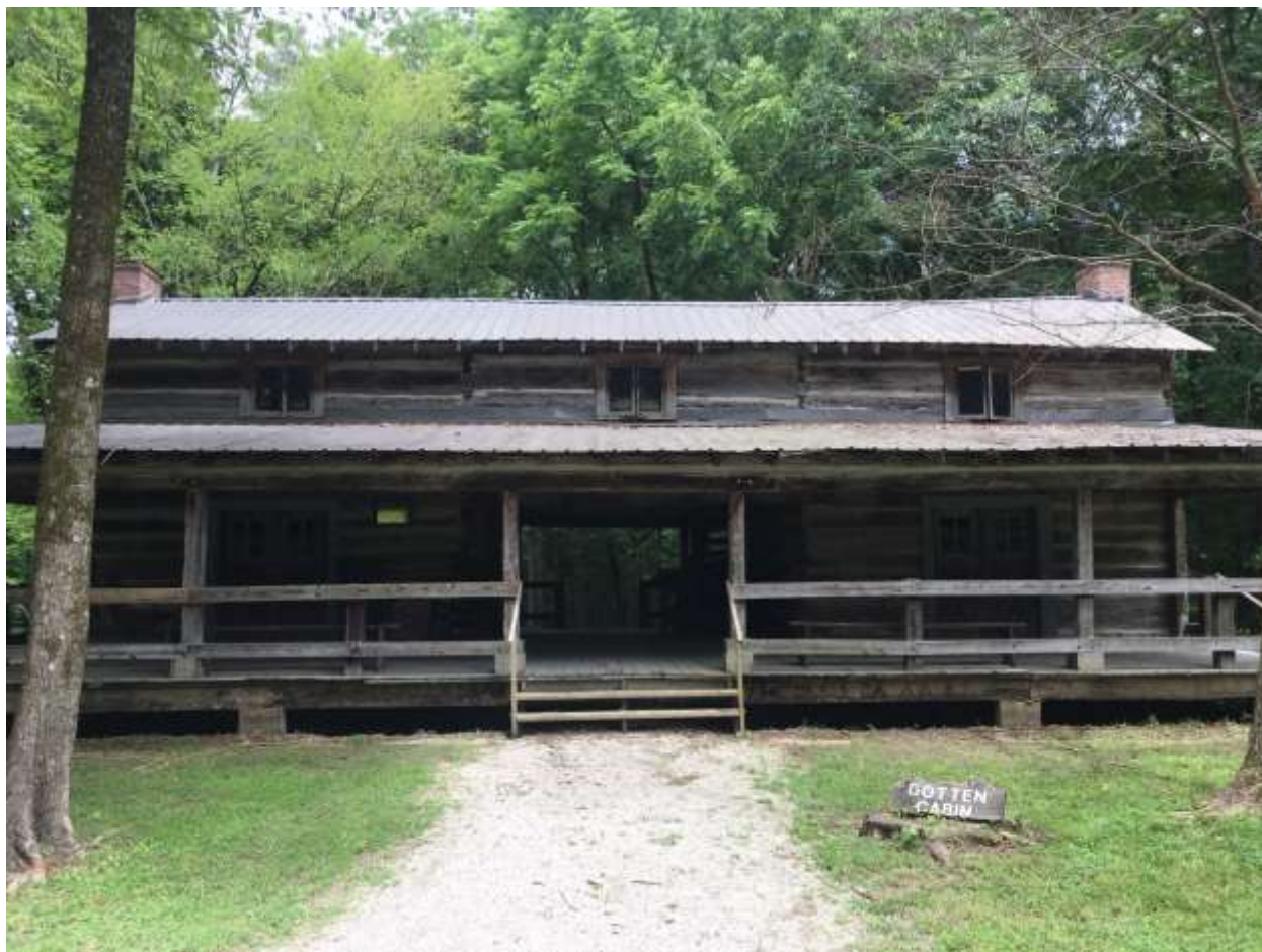
Figure 1: West-facing façade. Photo by Andrew Ross.
