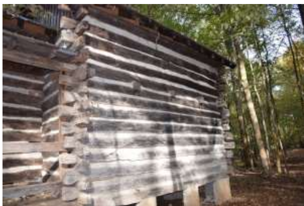
Figure 5: Loft joists seen from the exterior of the building.
