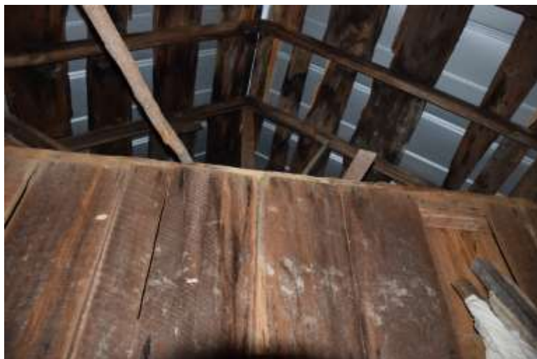
Figure 12: Stick-framing of roof as seen from the storage room.
