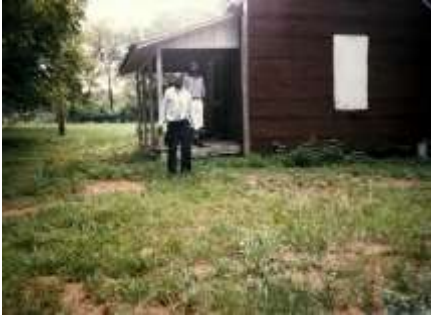
Figure 4: Asphalt siding on Mose's Cabin, late 1990s.
