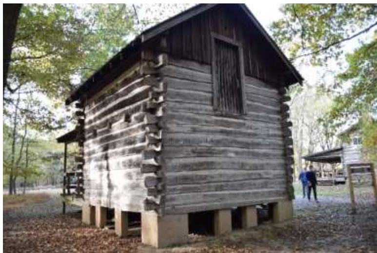
Figure 3: East façade showing upper-story and board-and-batten gable siding. South entryway to far left in background.
