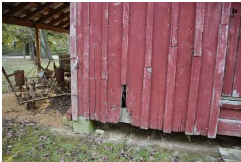
Figure 8: Exposed outer sill showing use of milled, dimensional lumber.
