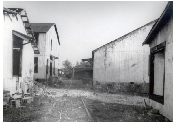
Cannonsburgh site before construction
