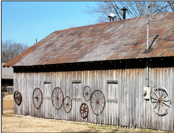
Blacksmith Shop roof
