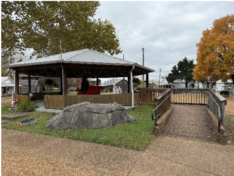
ADA-compliant Ramp on North-West Elevation
