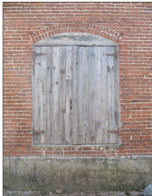
Cotton warehouse doors
