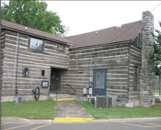
Visitor Center roof
