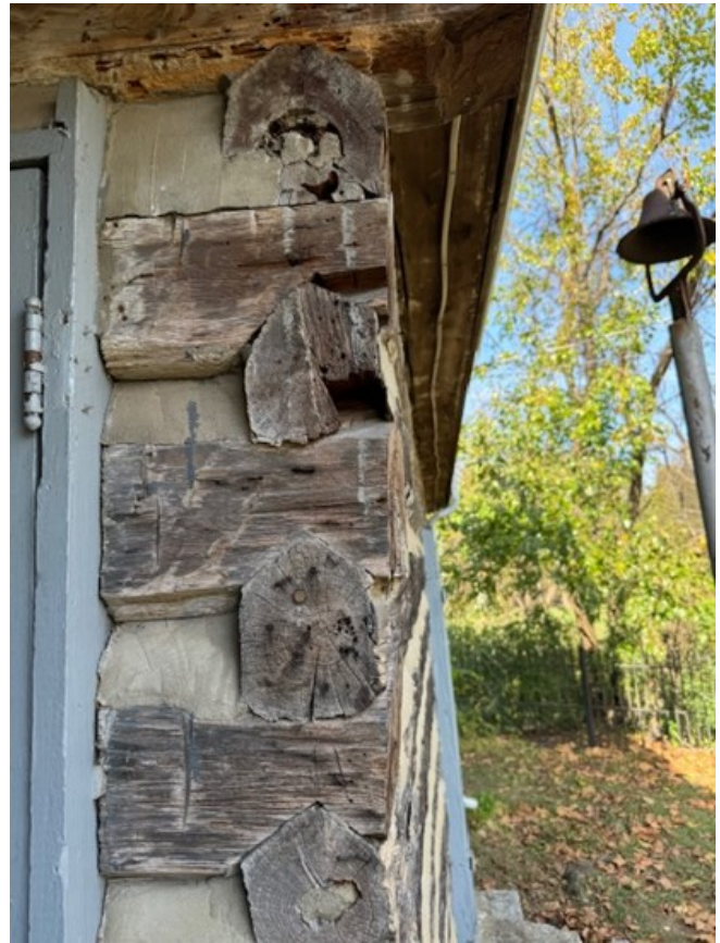
V-Notching with Holes, Southeast Elevation
