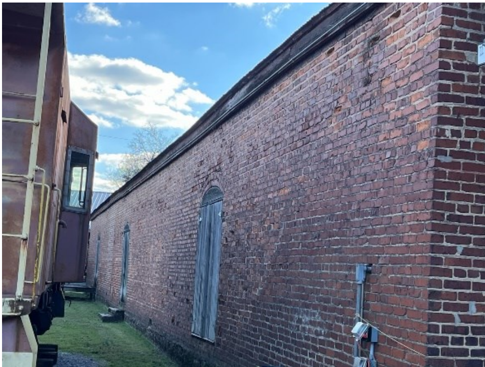
East Elevation Roof (No Gutter)
