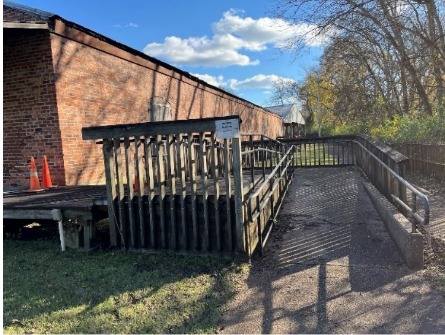
West Elevation ADA Ramp
