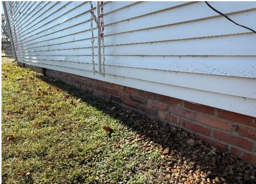
Brick Foundation Along East by Southeast Elevation
