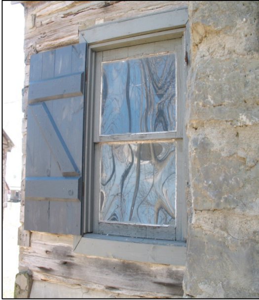
Town hall window and shutter
