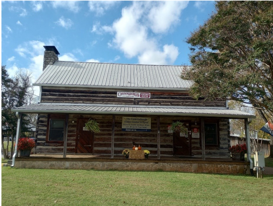
Visitor Center & Gift Shop, Northeast Elevation
