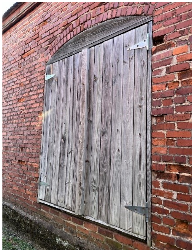
East Elevation Wood Doors
