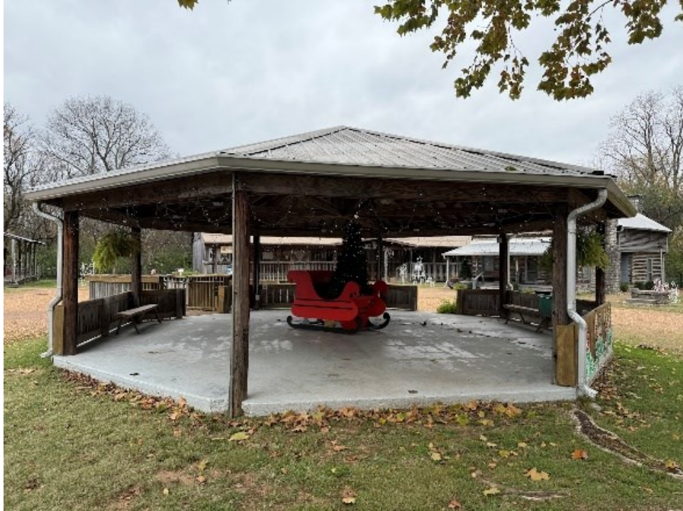
Pavilion on South-East Elevation
