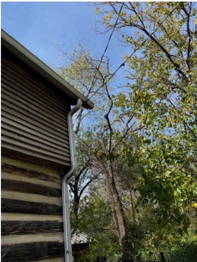
Exposed Romex Wiring, Southeast Elevation
