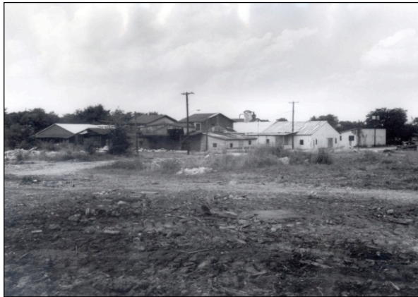
Cannonsburgh site before construction
