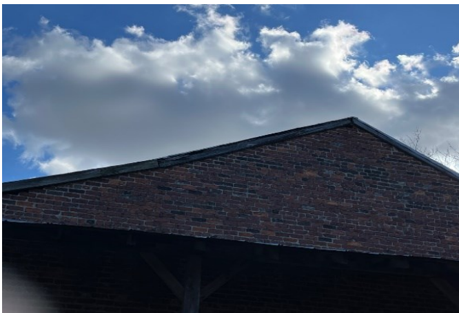
Roof on North Elevation
