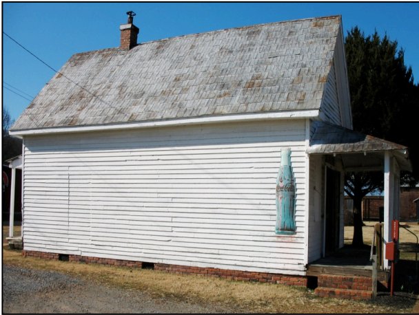
General Store roof
