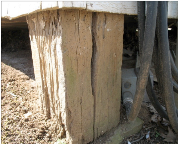
Wooden foundation at Telephone Exchange.
