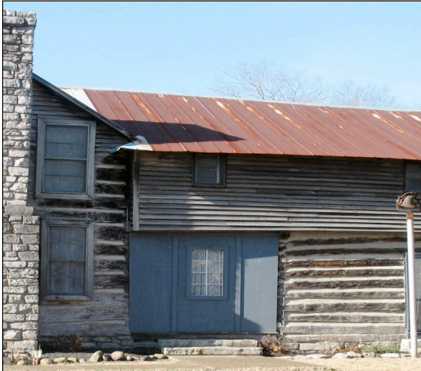
Leeman House roof
