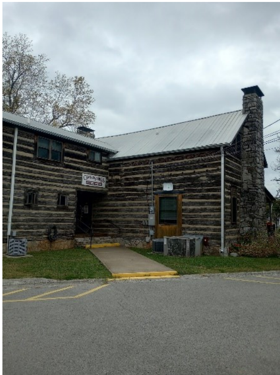
Southwest Elevation: HVAC System Visible
