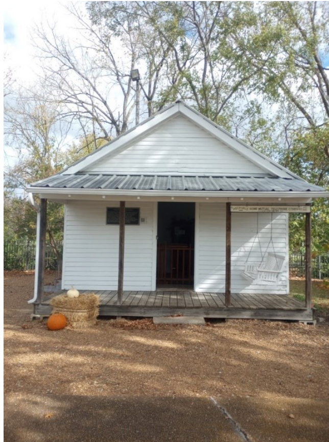
Telephone Building South Elevation
