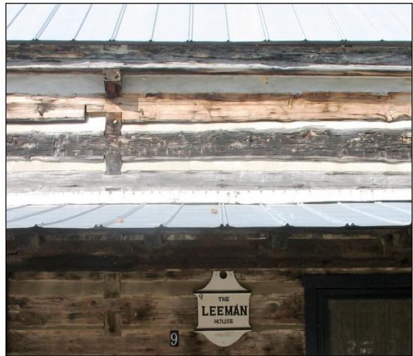
Aluminum flashing on Leeman House porch.
