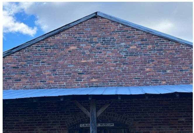
Porch on North Elevation
