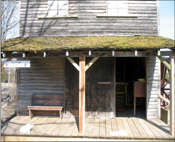
Grist mill porch roof
