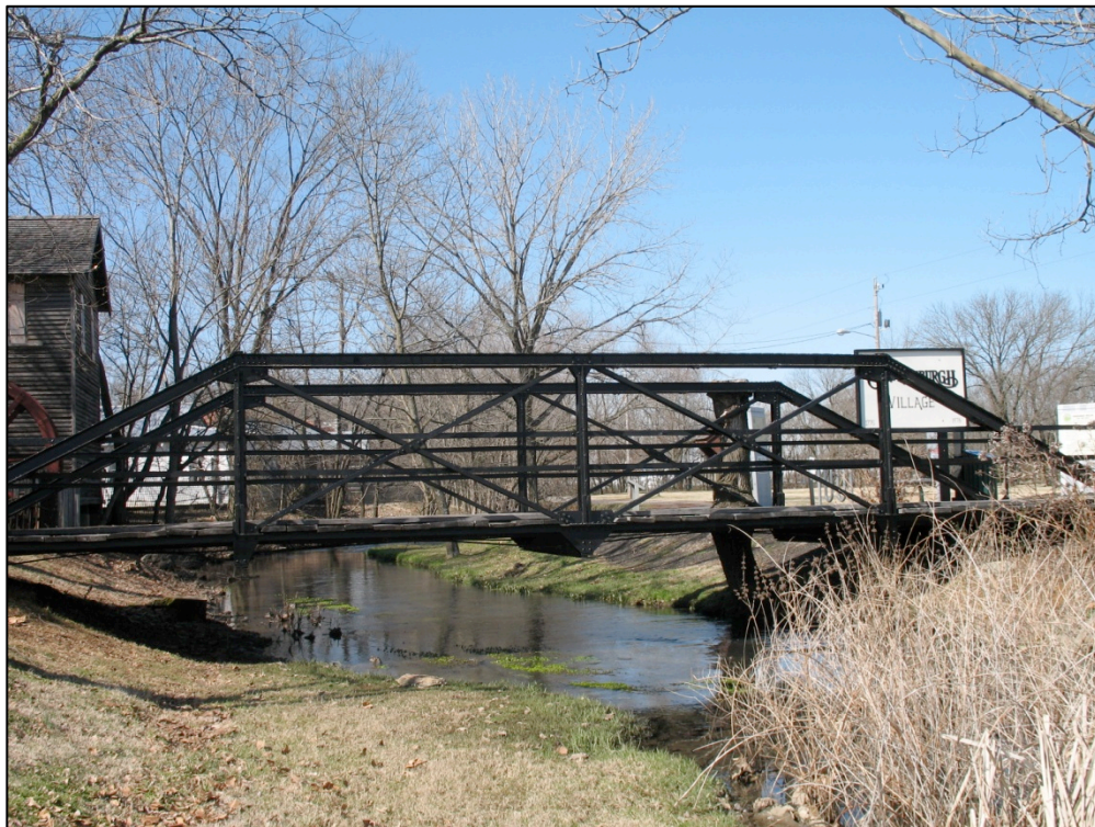
Toll bridge over Town Creek
