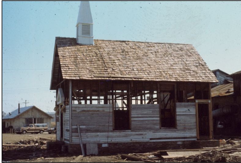
Williamson Chapel under construction in 1975.
