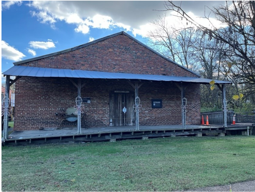
Cotton Warehouse North Elevation
