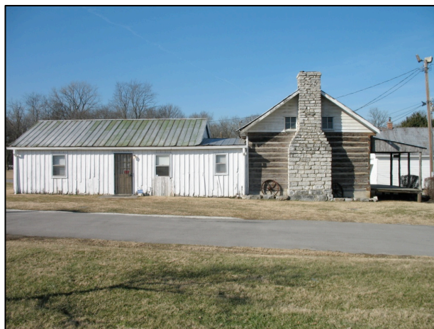
McKnight House linked to the storage building
