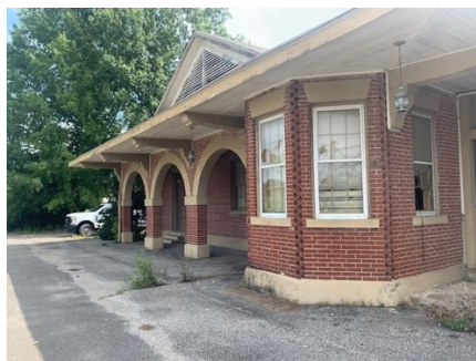
Trenton Railroad Depot
