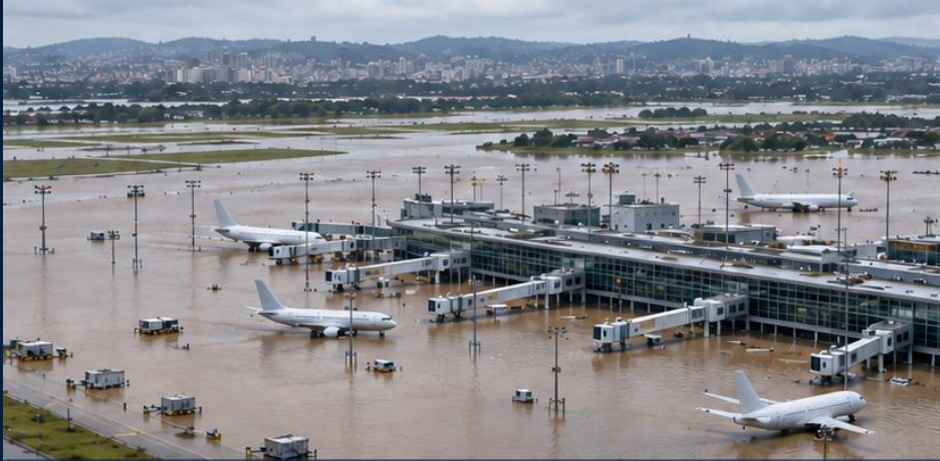
PORTO ALEGRE — AIRPORT FLOODING
