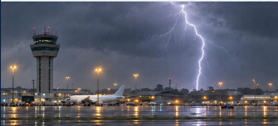
BRISTOL — THUNDERSTORM DAMAGE
