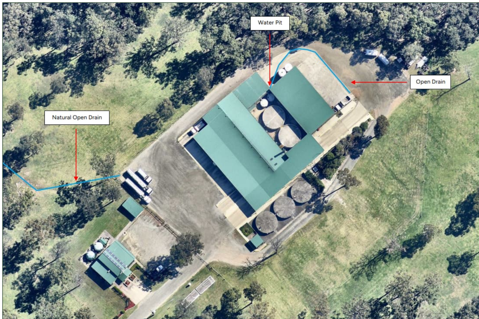
Figure 3: Location of Stormwater Drain on the Premises
