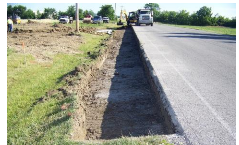
Road Widening Project
