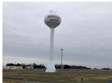
Pandora Water Tower
