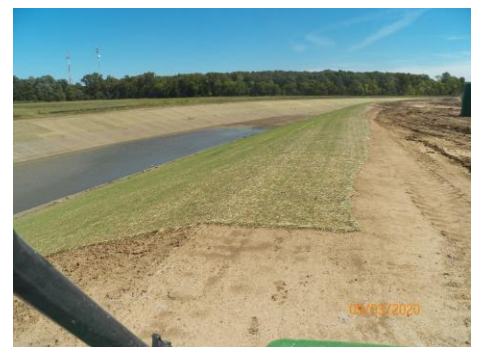
Ottawa Blanchard River Diversion Channel
