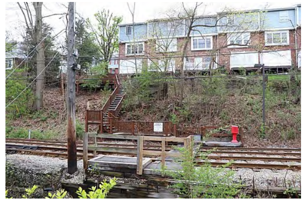
Sandy Creek Station
