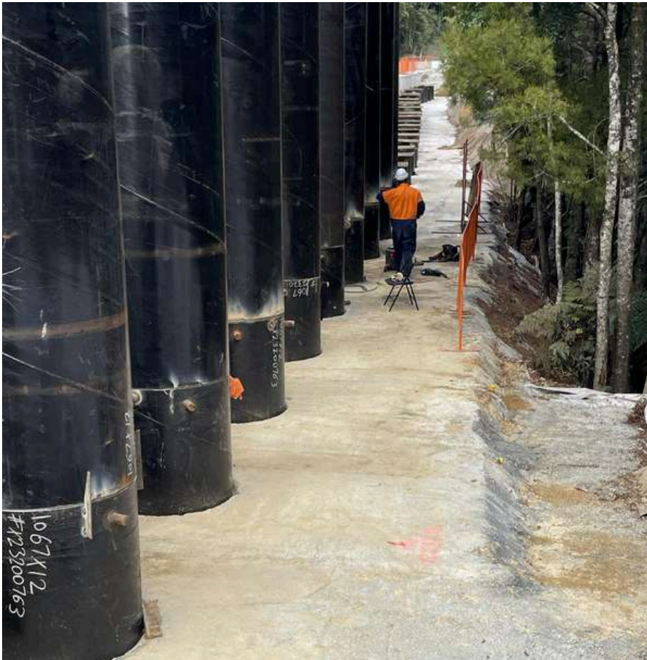
Slip A6 – Night works drilling piles in preparation for the day team to install the reinforcing cages.
