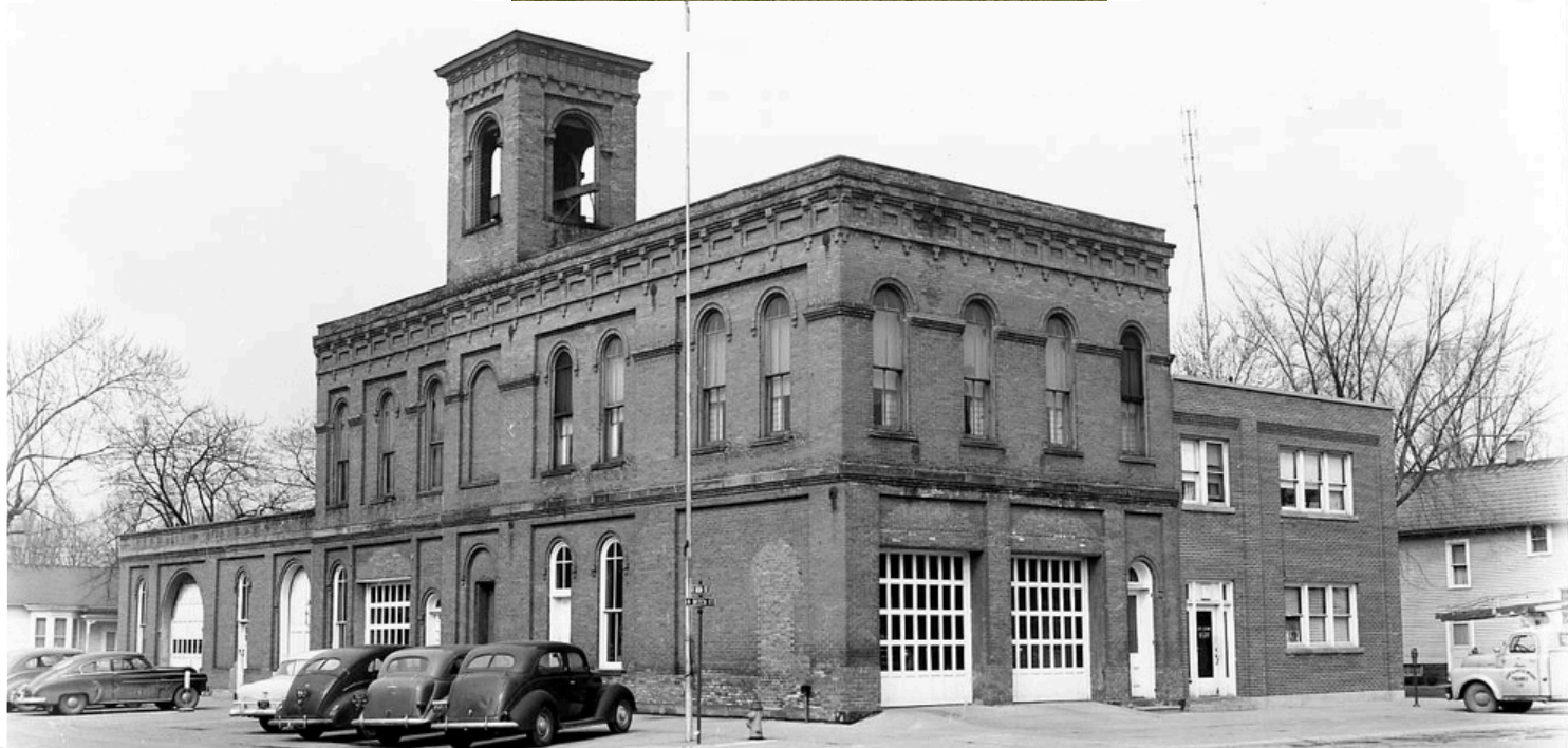
Photo Location: Fire Department
