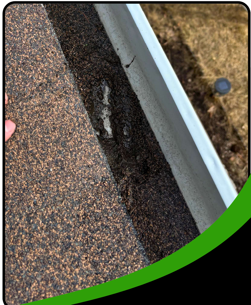
Granular loss in gutters
