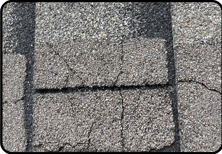
Exposed Fibreglass
