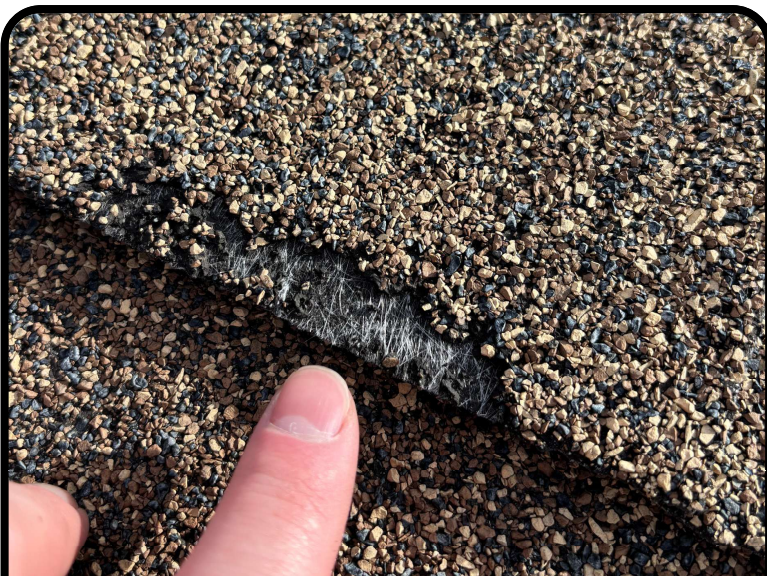
Exposed Fibreglass
