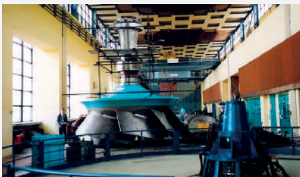
Deriaz turbine installation, Liptovská Mara PSHP
