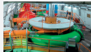
Francis unit: Before and after RMU Rama HPP, BIH; 100 MW, 2 units
