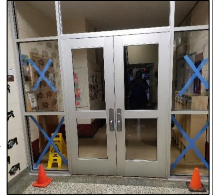
Installation of new door in progress
