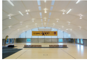
Tensioned ceiling - Sports hall (NZ)
