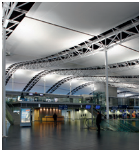
Tensioned ceilings Large flat or curved, continuous surfaces Quick installation and removal
