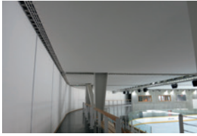
Ceiling & walls - Vaujany ice rink (FR)
