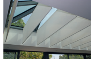
Ceiling & baffles - Restaurant (FR)
