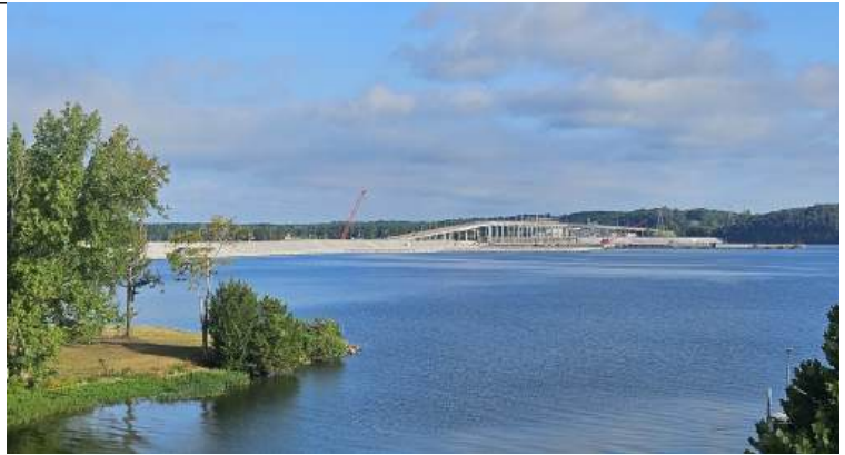
View from the hotel of the Pickwick Lake and Dam
