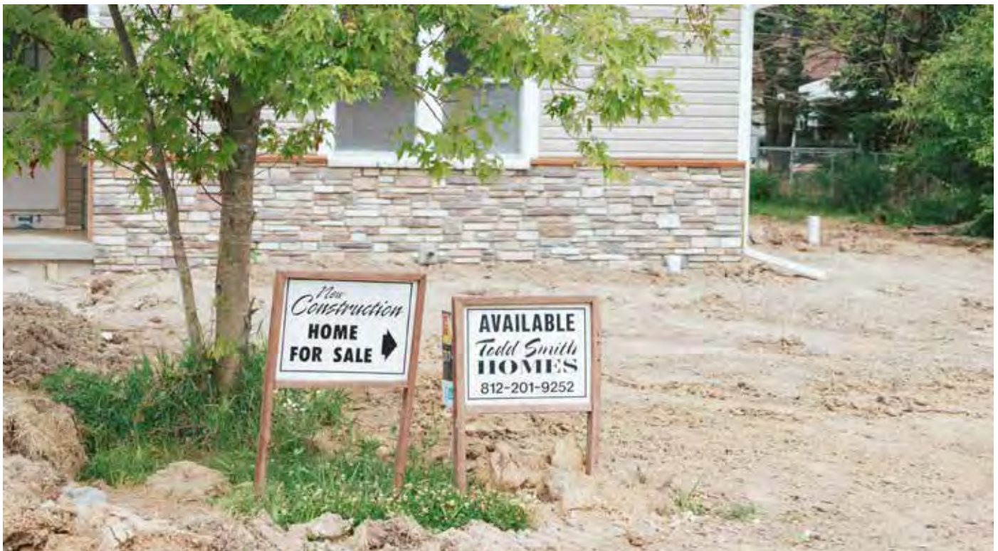
Signs point visitors to newly constructed homes at Heritage Lake. To keep up with growth and development in the area, the Clear Creek Conservancy District is upgrading its wastewater treatment system.
