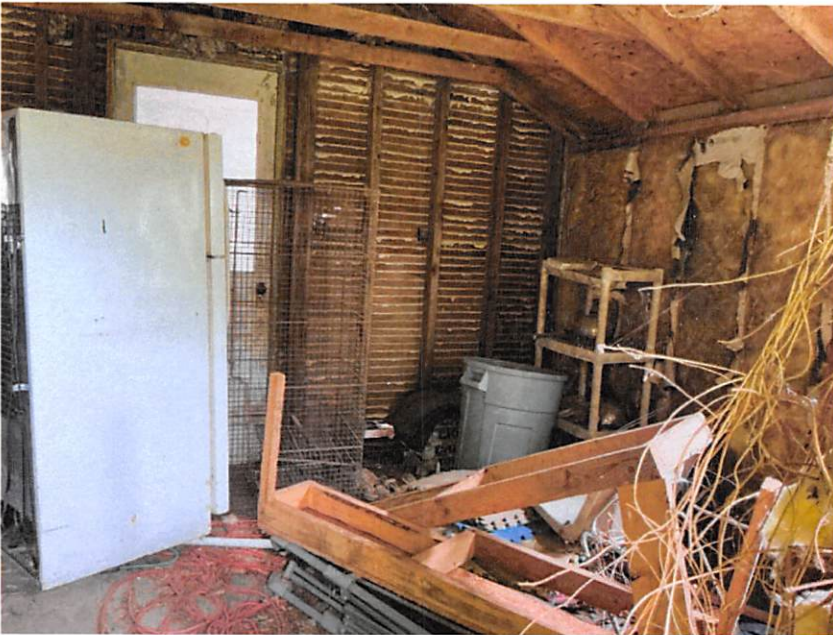
Inside of the structure -as seen through openings in the structure
