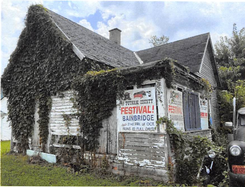
Different angle of dwelling as seen from Indiana Avenue
