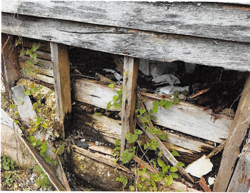
Missing siding/hole in dwelling
