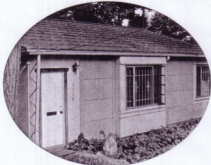
A wave of the future that never quite made it to shore, the Lustron porcelain-steel house was a factory-produced answer to the housing crunch packaged in a basic gable-roof dwelling. This Arlington, Virginia, model is among some 2,000 extant examples.
