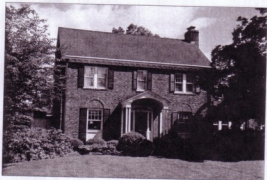
A full Colonial Revival of the era might look like this house built with Flemish bond brickwork and a neat entry porch with elliptical arch. Note the blind arches over the first-floor windows and the paired windows above them.
