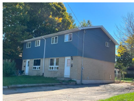
View of a completed siding replacement project
