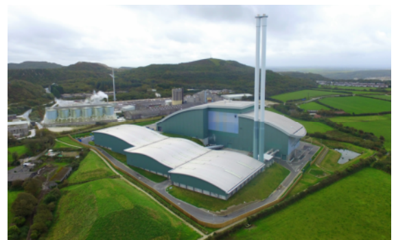
- Cornwall Energy Centre, St Austell
