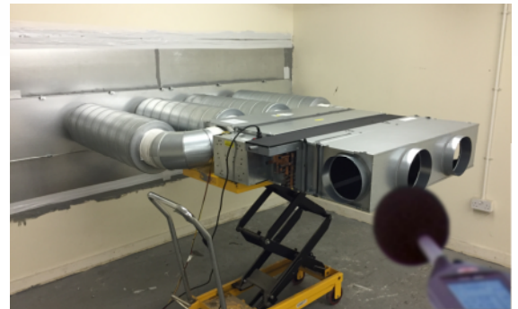
- Fan coil acoustic testing
