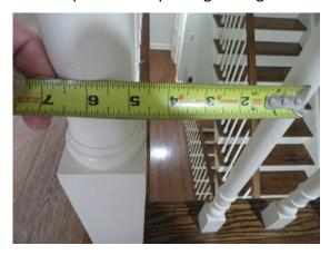
The handrail on at least one of the stairways is too low. It's about 32 inches but should be at least 34 inches. Another rail does not reach to the top of the stairs.
