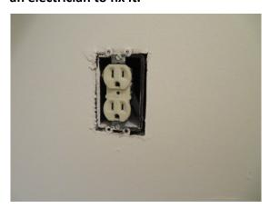
**16.** There is no ground fault circuit interrupter (GFCI) protection for the receptacles serving the kitchen countertop, outside receptacles, garage, and some bathroom countertops.
