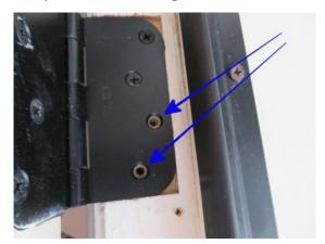
5. The hinges on the fence gate, leading to the kitchen exterior entrance door, are badly corroded. The force needed to open this gate is nearly enough to pull the gate hinges out. **Get a carpenter to replace the hinges.**
