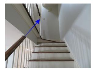
One of the stairway handrails is, by design, very loose.
