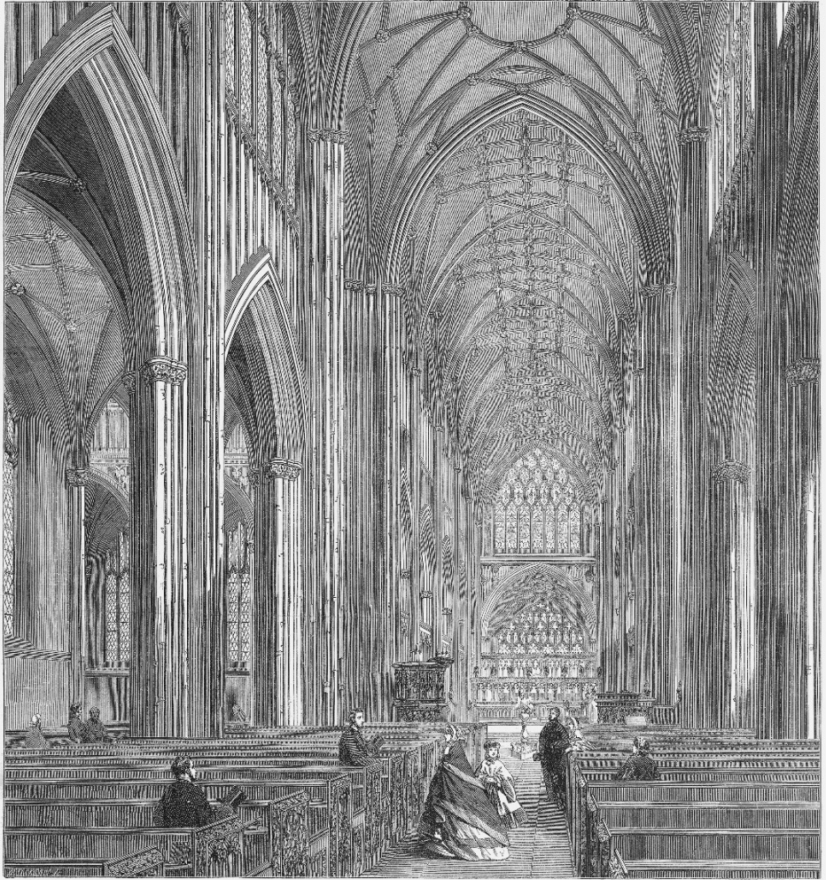
ST. MARY REDCLIFF, BRISTOL, IN PROCESS OF RESTORATION UNDER THE DIRECTION OF MR. G. GOWNS, ARCHITECT.
