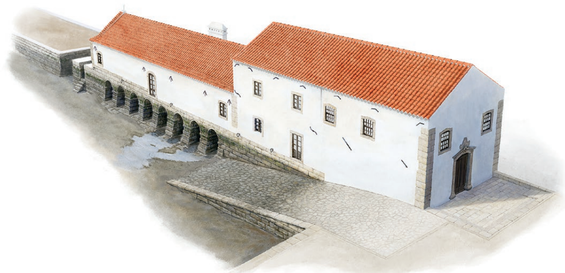
Figure 3: (above) The Corroios tide mill, with the distinctive eight arches that house the milling mechanisms.
