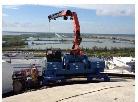
using wire rope cables and rigging hardware. Two additional cables secured the vent stack to the building. The new structure had the dual function of supporting the vent stack in hurricane wind conditions and serving as a safe, secure work platform in operating conditions.
