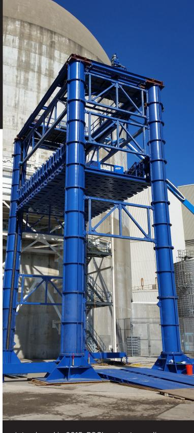
Introduced in 2015, PSC's patent-pending PIPE MODULAR LIFT SYSTEM (PMLS) eliminates the hazards of suspended loads, elements of wind and reliance on cranes. The PMLS provides a safer and faster method to support elevated reactor building equipment hatches.
