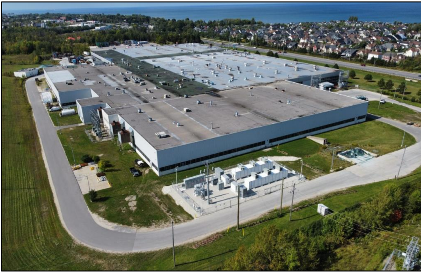
Pilkington BESS (5 MW / 10 MWh), Collingwood. Operational since 2022.
