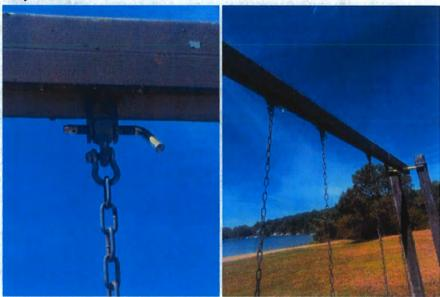
**Comments** Play structure is using receiver pins that are missing
