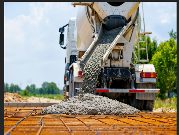
Figure 1: This research shows the tradeoff of standard load vs. fully-loaded RMC trucks, finding that the latter enables 32.5% lower fuel consumption and 5.6% truck-pavement system cost savings, while having comparable impacts on pavement deterioration.
