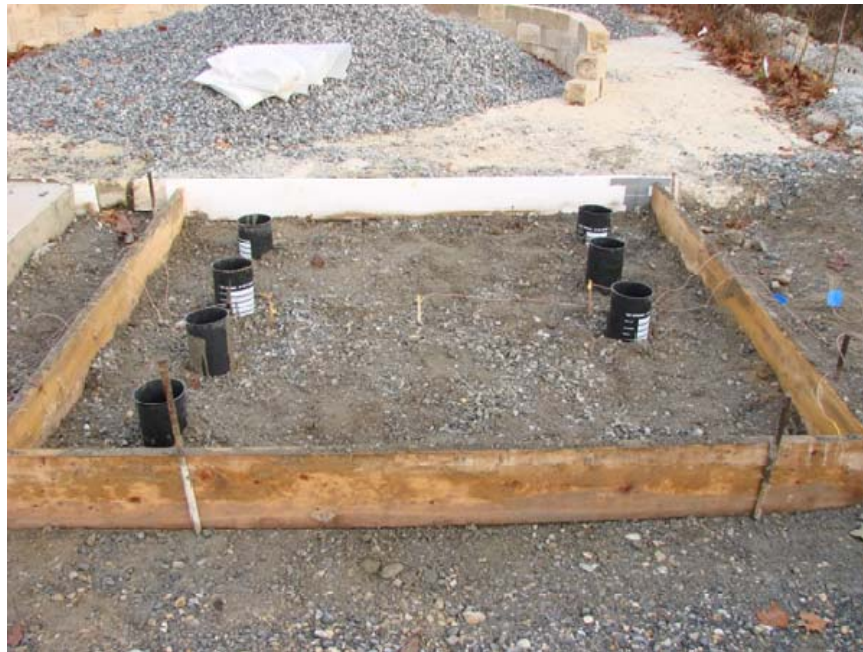
Figure 4.7 Concrete slab with cast-in-place cylinders and temperature sensors
