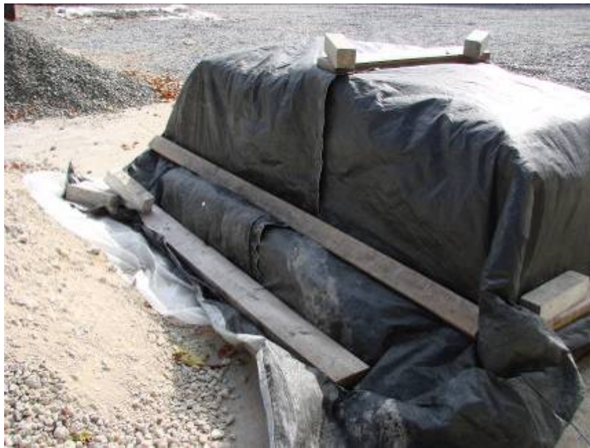
Figure 4.6 Concrete block curing in field.
