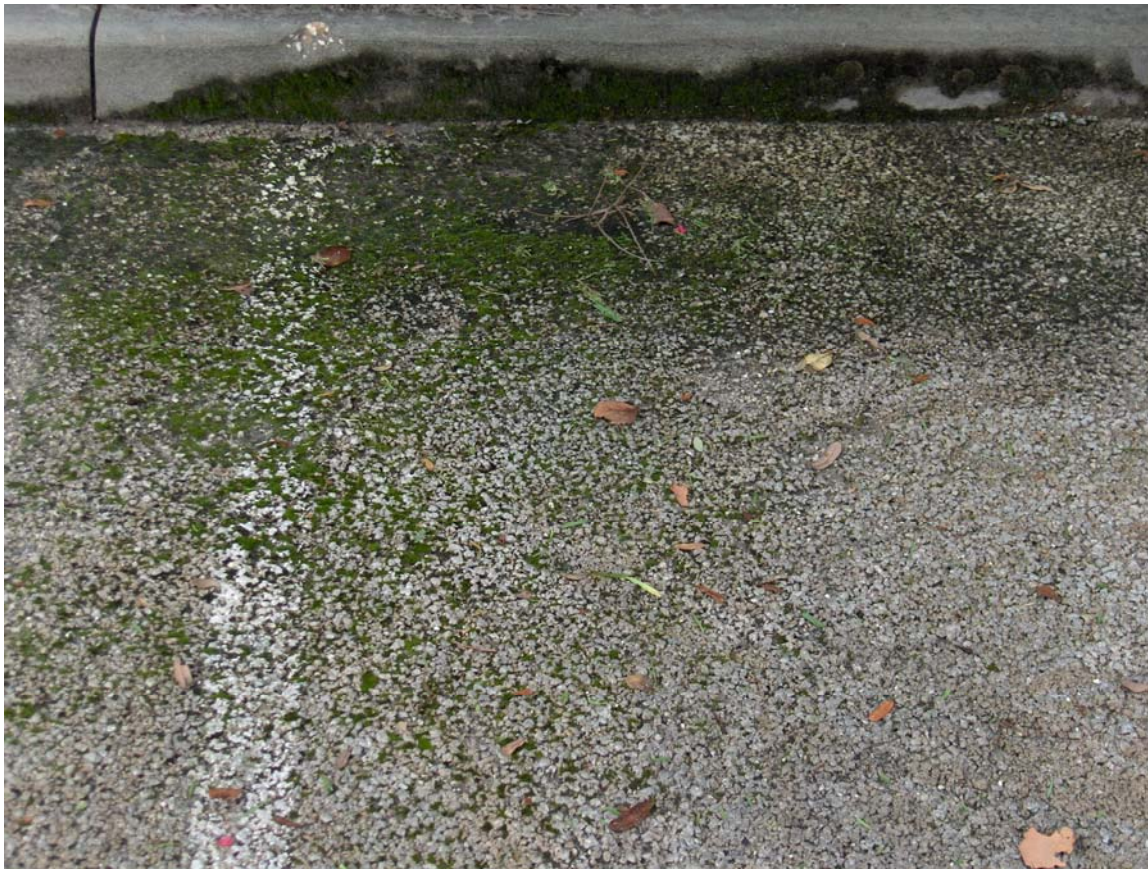
Figure 24: FCP&A Parking Lot
