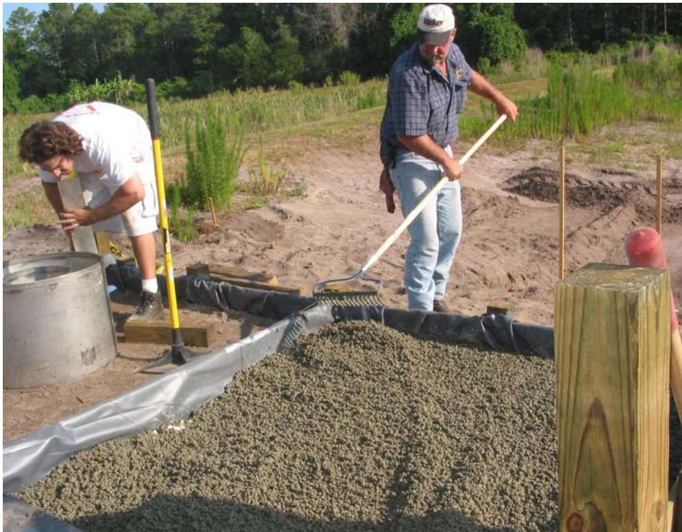
Figure 3: Stormwater Academy Porous Concrete Test Cell Installation
