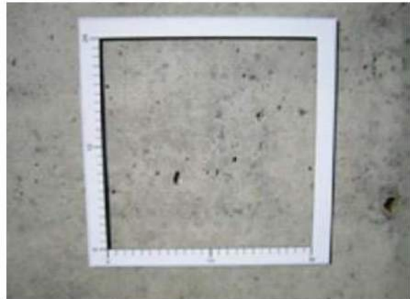
Fig. 3.2a(c)—Close-up view of wall Fig. 3.2a(a) at a different location.
