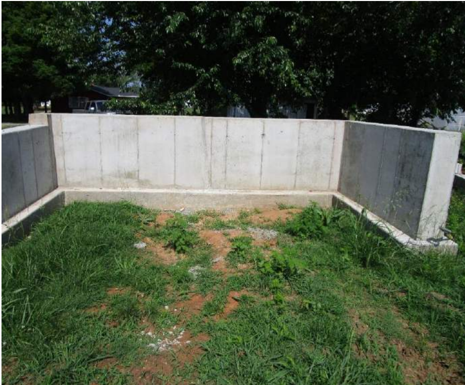
Fig. 6.5 MTSU test wall immediately after form stripping and six weeks later
