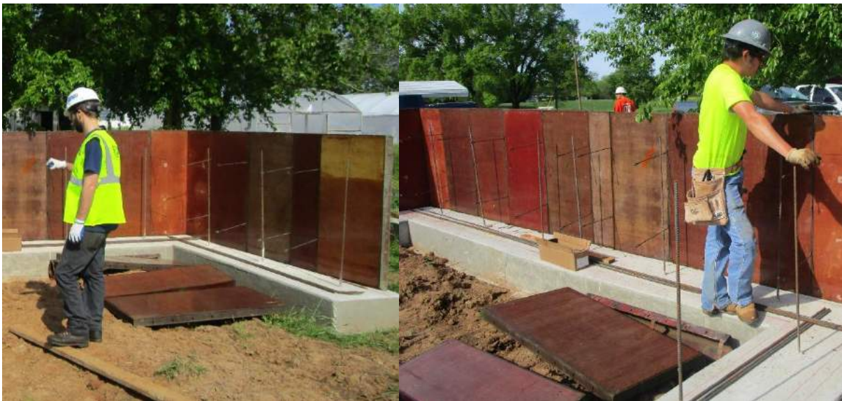
Photo 2. N and W outside wall forms
