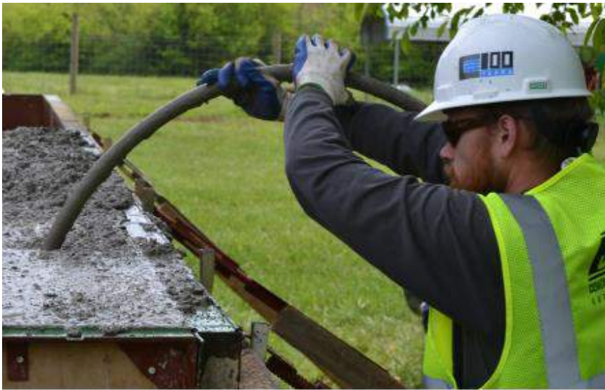
Photo 6. Vibration with a 2-in.-diameter internal vibrator
