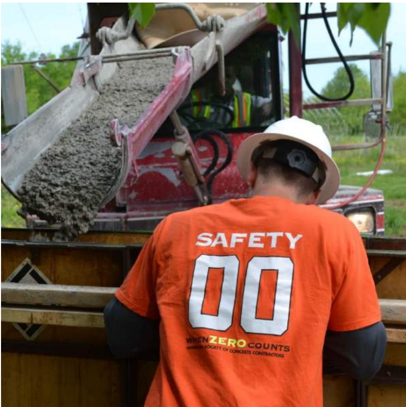
Photo 5. Concrete placed in the forms from a front-discharge truck.
