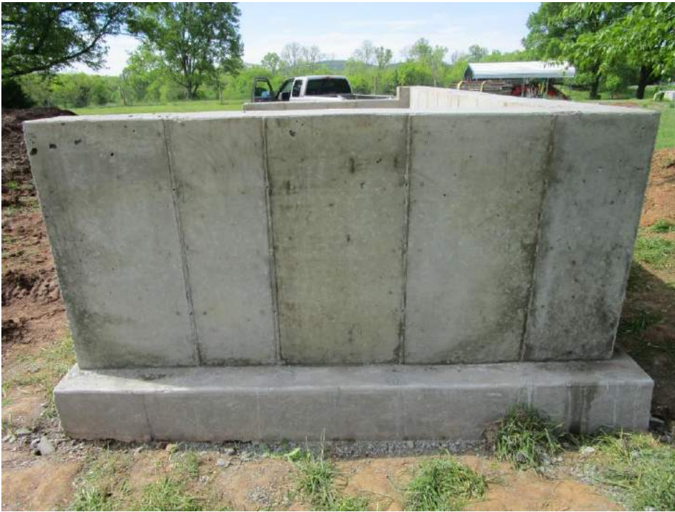
Photo 7 Outside face, north wall on day forms were stripped
