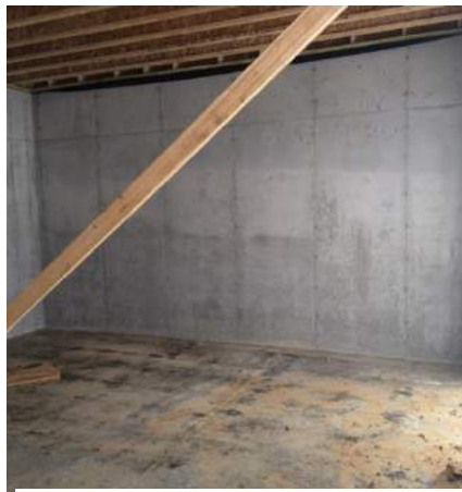
Small residence inside wall
