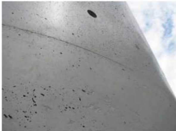
(a) General view of formed surface with high ratio of surface voids and imperfections
