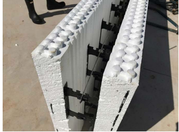
Image 10: Example of a typical ICF block
