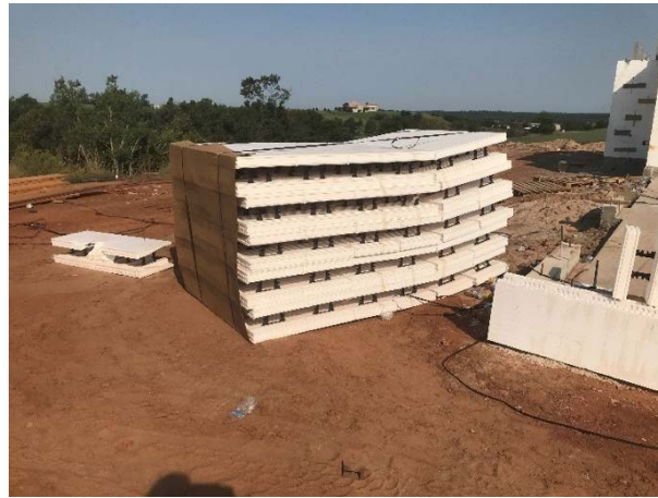
Image 11: Example of a shipment of ICF blocks on the jobsite
