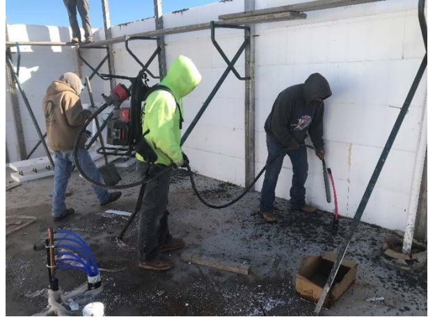
Image 6: Workers vibrate the concrete inside the ICF walls
