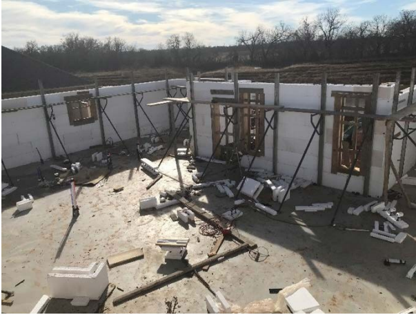
Image 5: View of inside of ICF house prior to concrete placement
