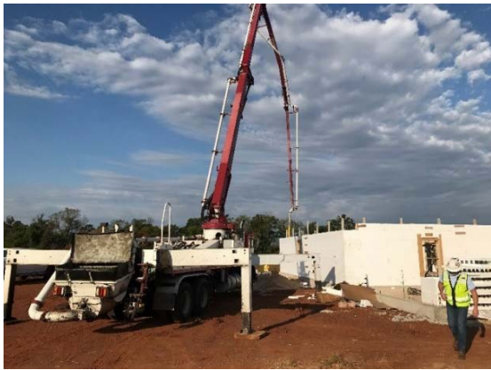
Fig 2a – ICF installed courses to form the wall Fig 2b – Concrete poured using pump truck
