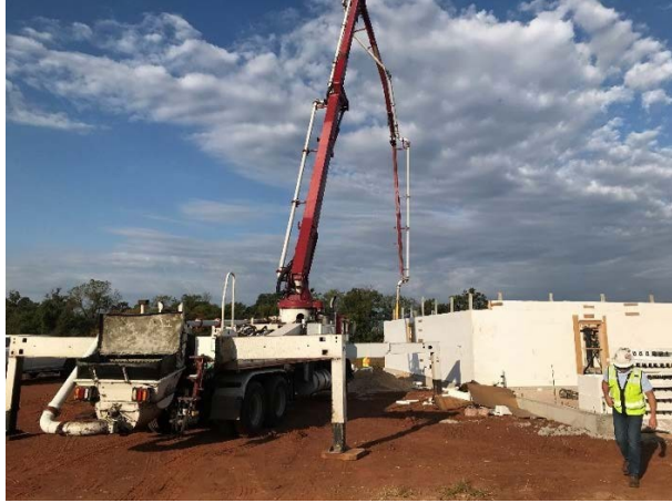
Image 7: Pump truck at ICF house site
