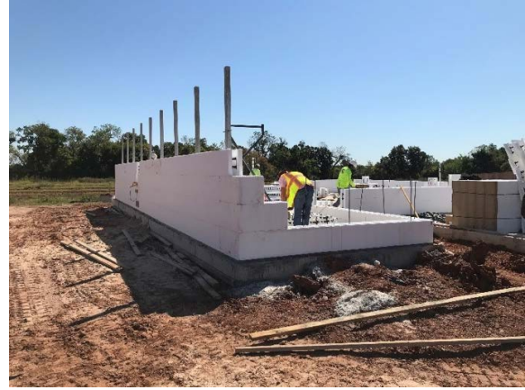
Image 4: Workers install courses of ICF blocks
