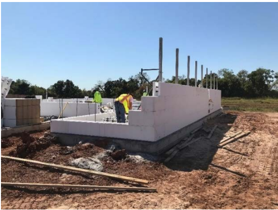
Fig 2a – ICF installed courses to form the wall Fig 2b – Concrete poured using pump truck
