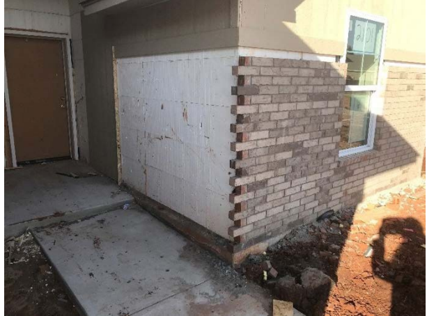
Image 8: A view of ICF blocks before final exterior cladding is installed
