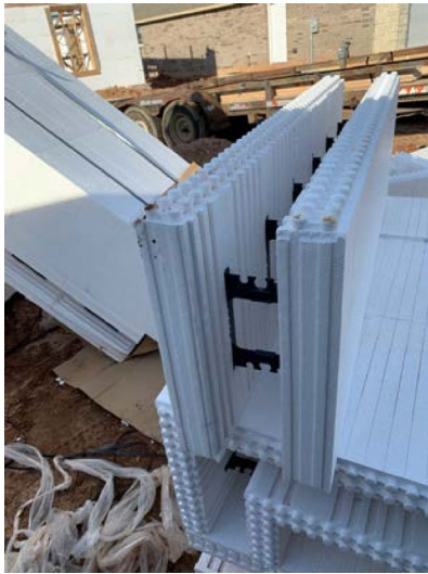
Fig 1a – ICF block used in the houses
