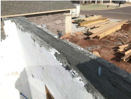
Fig 2c – Concrete filled ICF wall
