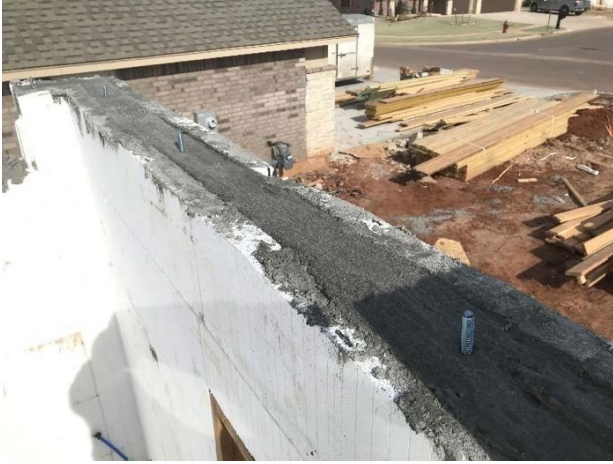
Image 9: A view from the top of ICF filled with concrete
