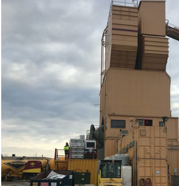
Figure 1: Centralized Batching and Mixing
