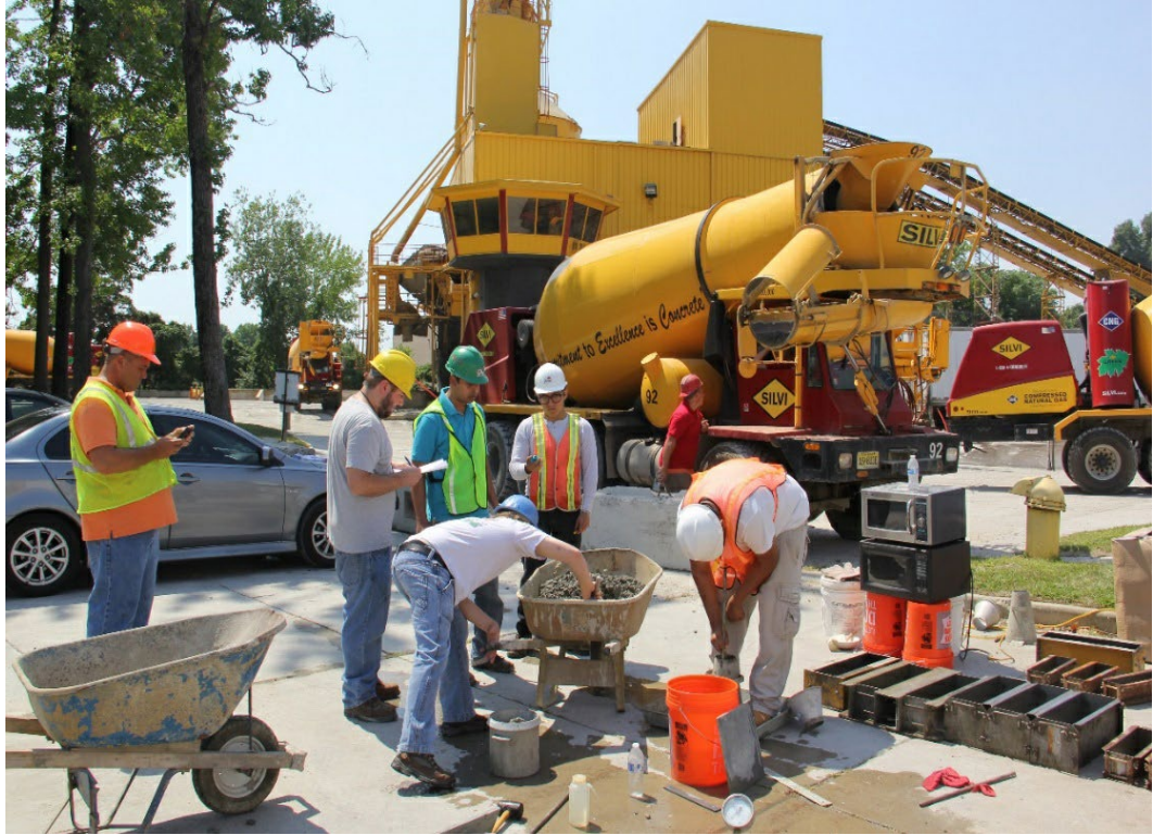
Figure 2: Slump and Air Content Test in Progress
