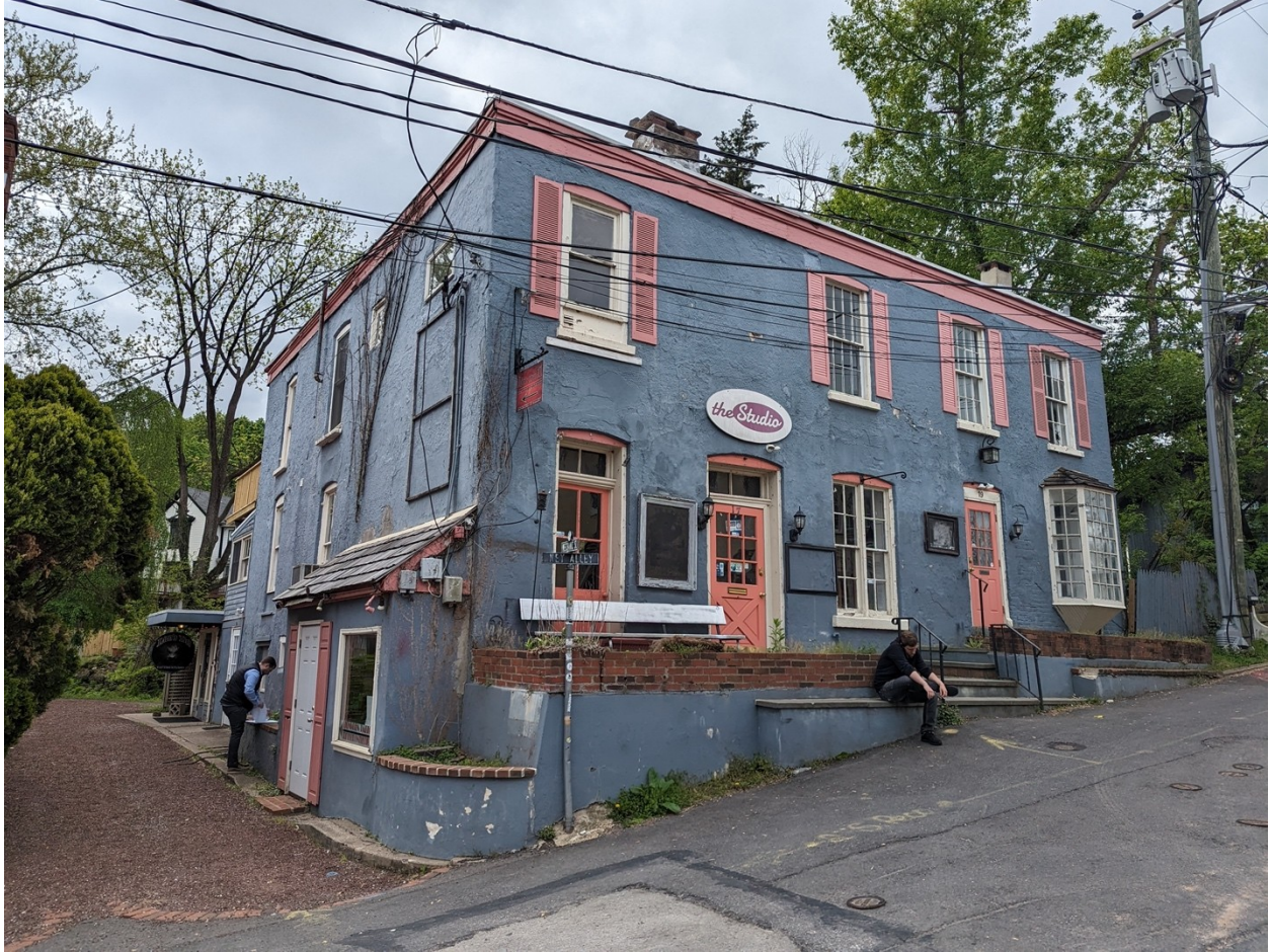
Subject structure prior to most recent renovation.
