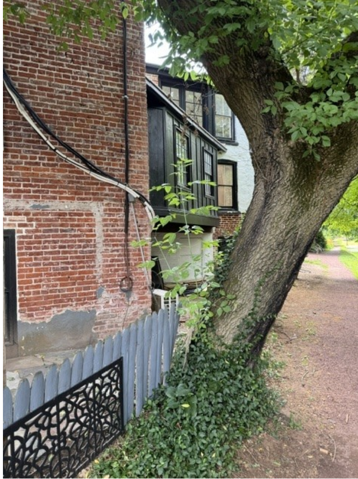
Rear of building along the canal Towpath.
