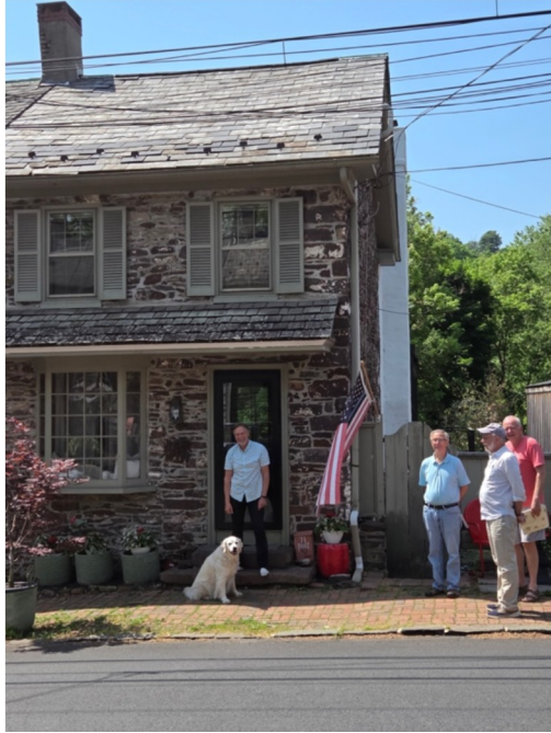
71 W Ferry St, owner Lou Bellafronte at door, and NHHS volunteers
