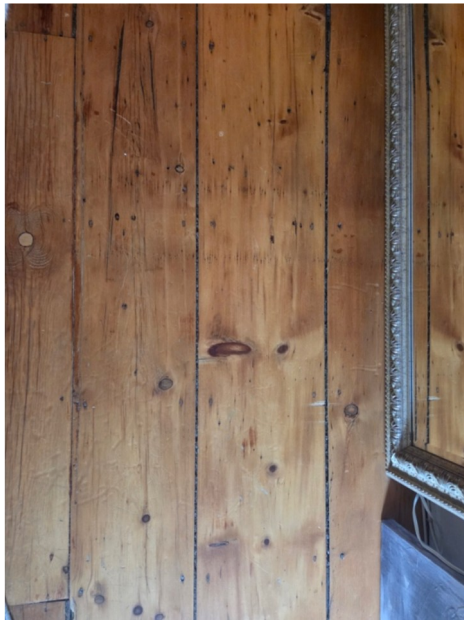
Original floors, 71 W Ferry St.
