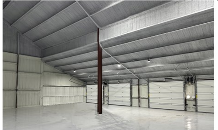
FS 2.0 completed on a multi-purpose metal building project
